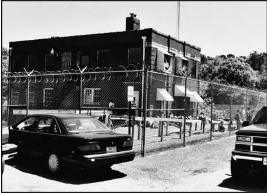
A view of jail property, hose drying rack
